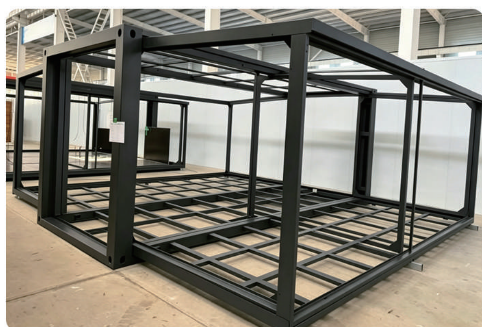
Reinforced Steel Structure Frame
